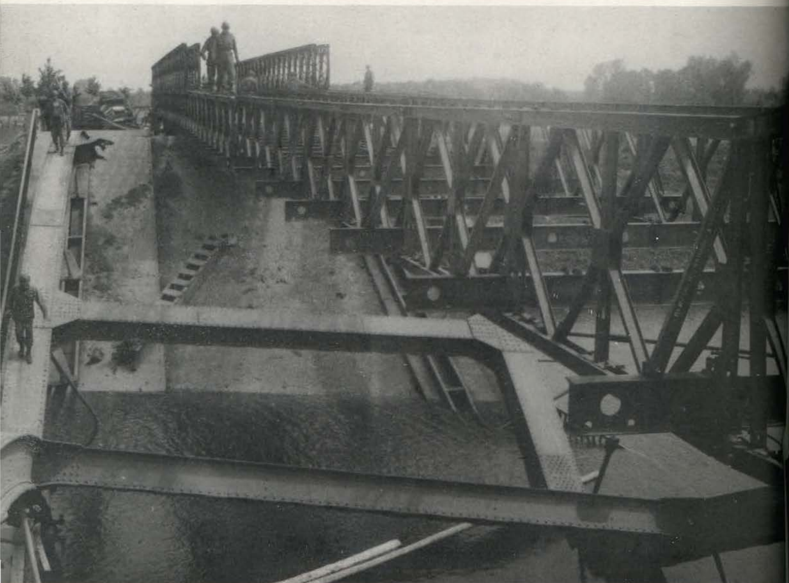
Members of the 320th Engineer Battalion throw a Bailey span across a canal above the remains of a destroyed German bridge.
