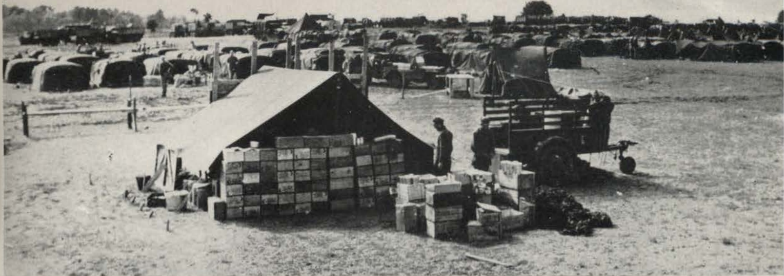
For many in the Division, driving six-ton loads of fuel and ammunition on the Red Ball express route to the American Third and British Second armies was their first taste of near-combat. This is the base camp of one of the provisional companies, near Gisors, France.
